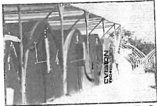
Figure 394. A Texas Reishi production facility. By modifying hoop-framed greenhouses and covering them with an open-sided, metal roofed super-structure growing rooms can be constructed at low cost.
