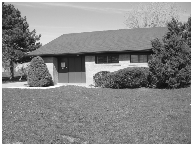
Figure 9.3 A covert electrical substation.
